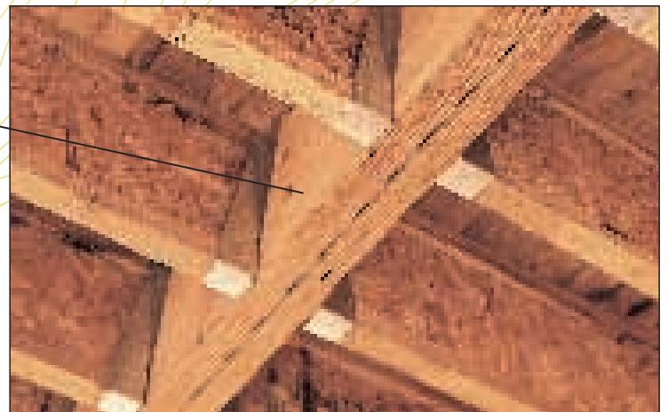
Laminated Veneer Lumber (LVL) being used with I-joists.
