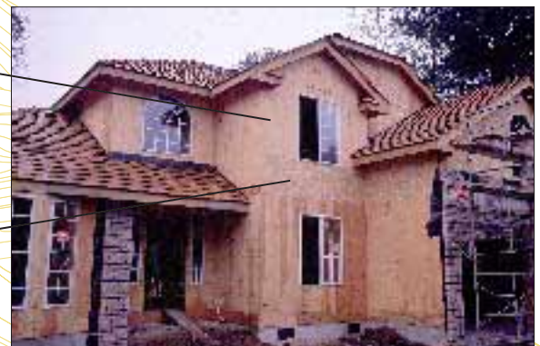
Structural Panels in their construction application.
